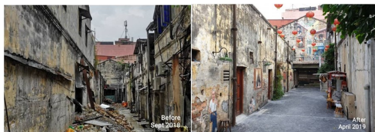
Figure 7: Before and after revitalization of “Little Demon Alley” Source: Bai Chuan Management
