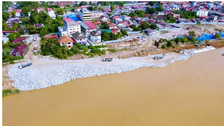
Figure 4: The Construction Progress
