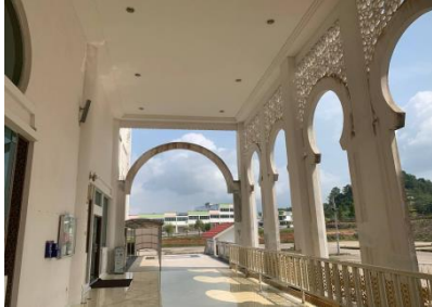
Figure 4. Defect: stagnant water Source: Authors (2024)
