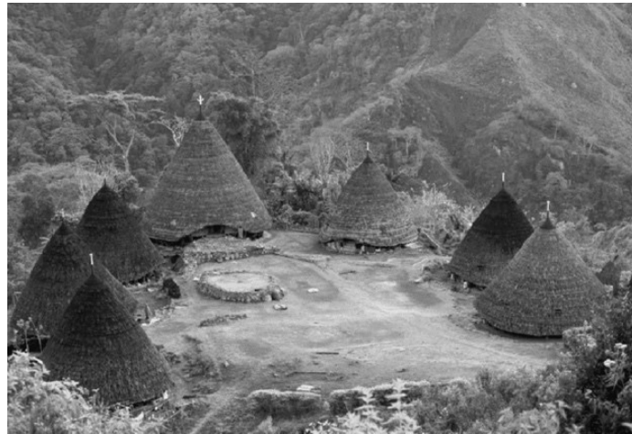
Figure 1: Example of Vernacular Architecture of Mbaru Niang shows the uses of local materials and is designed to suit the local conditions
