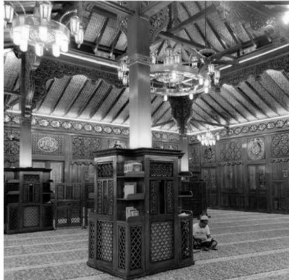
Figure 9: Installation of an air conditioner at the bottom of Soko Guru, and concealed and served as a bookshelf without compromising the traditional ambience
