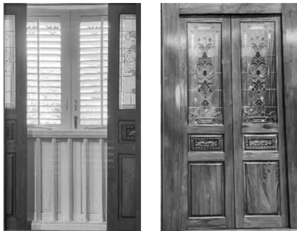
Figure 6: Retrofitting detailing on the window of Masjid Al-Qadim Source: Author
