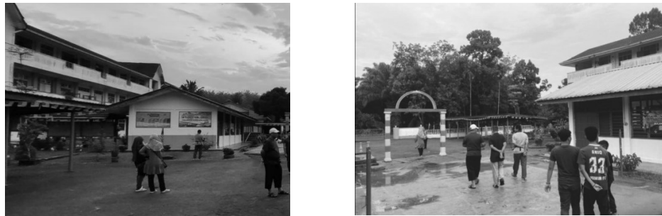
Figure 7: The current condition at SK Sg Kiol in Jerantut, Pahang.
