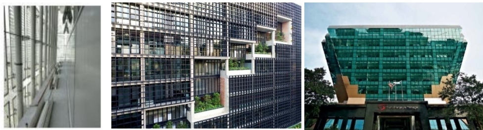
Figure 1: Selected high-rise office buildings in Malaysia used as case studies (Suasana PJH, PAM Centre, and Suruhanjaya Tenaga), illustrating the diverse application of passive facade strategies in tropical climates.
