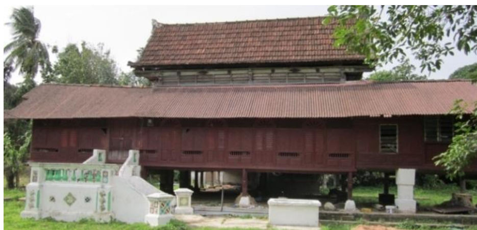
Figure 1 A Traditional Malay House in Rembau, Negeri Sembilan with an Attic Space
