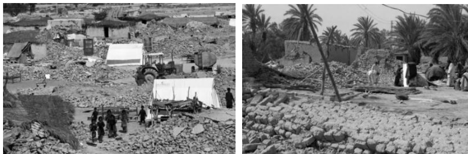
Figure 1 Earthquake damages in Awaran during September 2013
