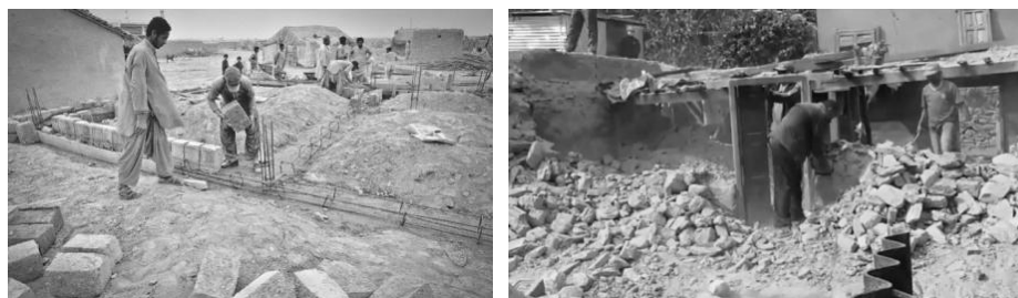
Figure 2: Housing Re-construction in Awaran
