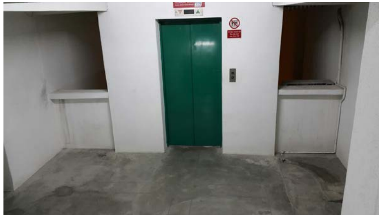
Figure 12: Under-utilised space: an existing lift lobby in an apartment
