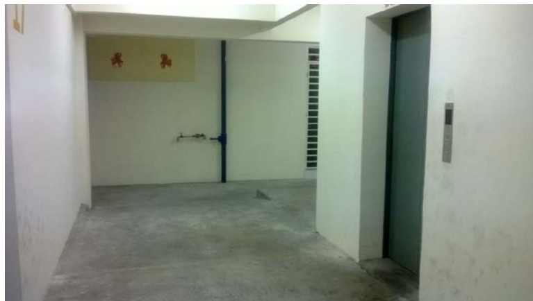
Figure 13: Under-utilised space: an existing lift lobby in an apartment
