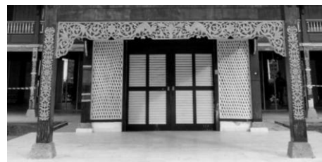
Figure 20: Most of Malay houses with pedestal called ‘lapik tiang’ (base of the post) or ‘alam tiang.’
