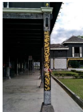
Figure 18: Columns and pedestals At Istana Seri Menanti, Negeri Sembilan
