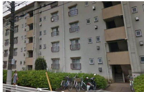
Figure 2: Stairs connecting apartment units in each floor in Oyamadai-danchi
