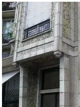
Figure 26: The decorative finials which similar to the buah buton Malay Asian timber based tradition.
