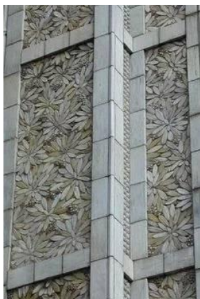
Figure 25: Perret's Rue D Apartment France, flower motifs used to decorate empty surfaces of concrete walls
