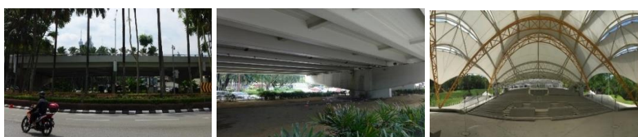
Figure 3: Lost spaces identified by the respondents. (i) Roundabout in Jalan Kuching, Kuala Lumpur; (ii) Viaduct of Jalan Kuching - Jalan Tun Perak; (iii) Pangung Anniversari
