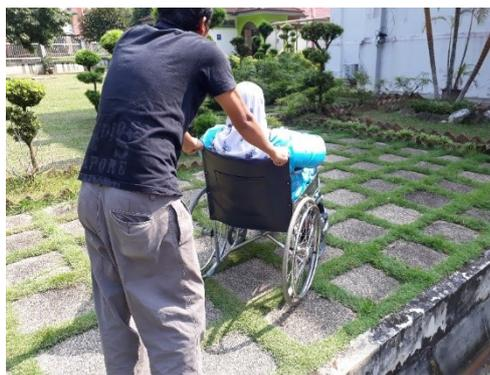
**Figure 3:** Unsuitable material used for the route to the accessible toilet
