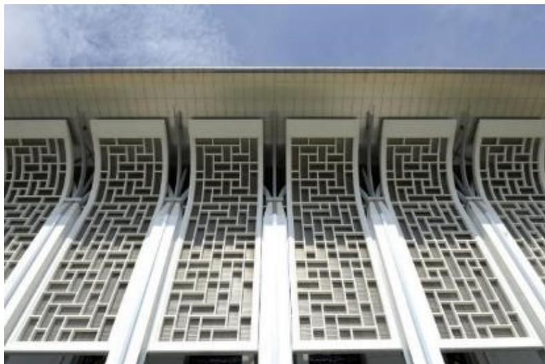
**Figure 12:** the stainless-steel spiral mesh at the back of the rectangular pattern
