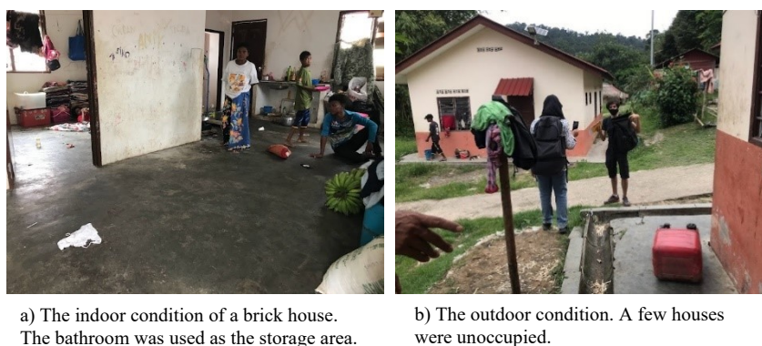
Figure 6: The condition of brick houses initiative by the government in Bongor
