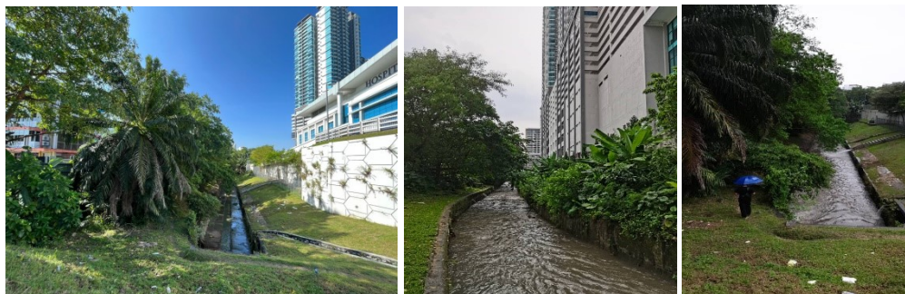
Figure 1: The existing condition of the proposal Linear Park and Community Garden Source: The authors
