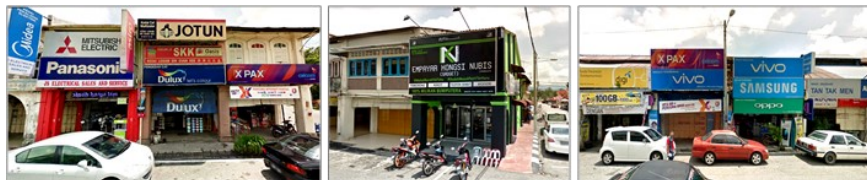
Figure 6: Improperly placed, oversized, and excessive signage disrupt façade continuity, streetscape harmony, and reduce the building's architectural aesthetic.
