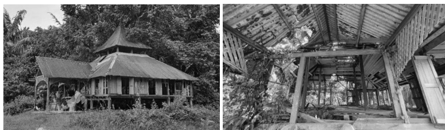
Figure 1: The actual condition of Masjid Lama Kampung Pelangai, Kuala Pilah. Sources: Author, 2024
